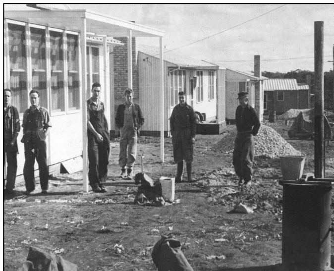
Jack Blythe (2nd from right) and workmates building houses in Newborough for SEC employees -1950
