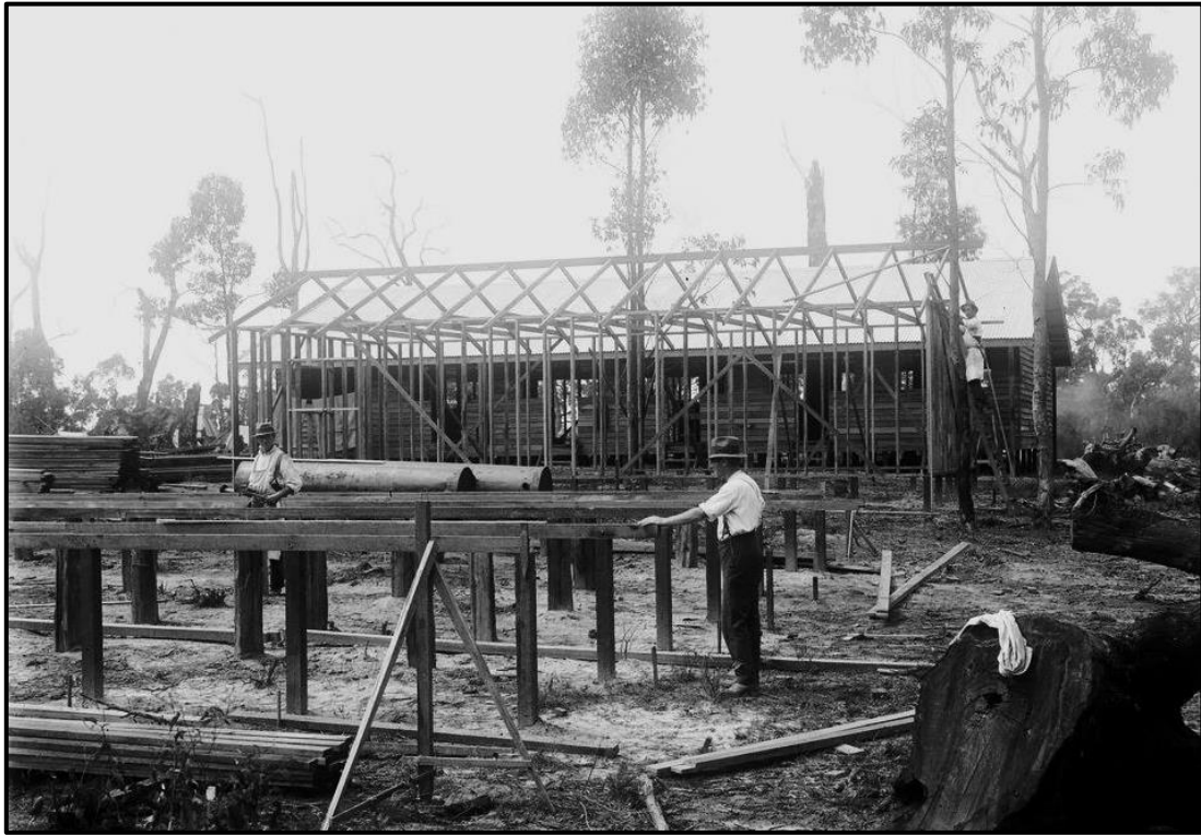
West Camp- Building of cubicles
