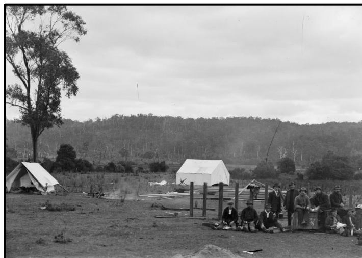
Eastern Camp when the temporary power plant was under construction.
