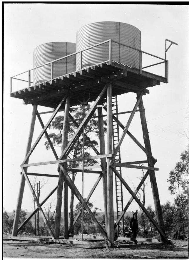
The water tower and tanks for the West Camp.
