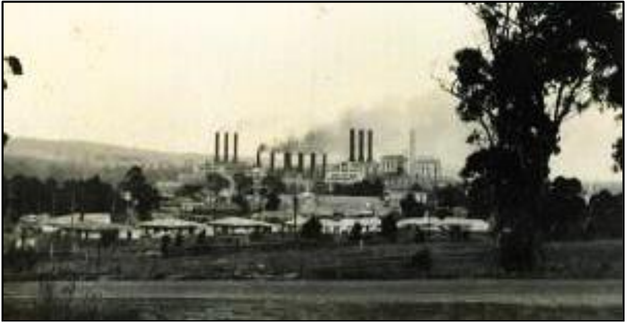
A section of the Married Quarters can be seen in the foreground of the photograph.
