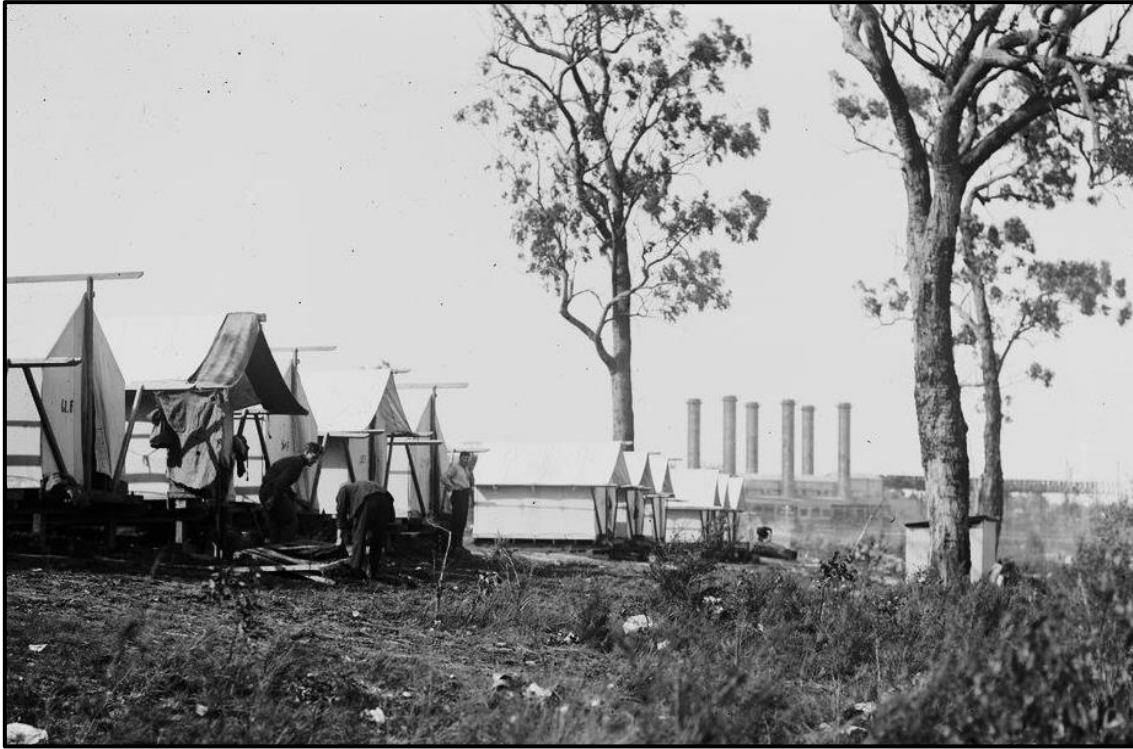
West Camp area. The power station can be seen in the background Source: H2009 18/280
