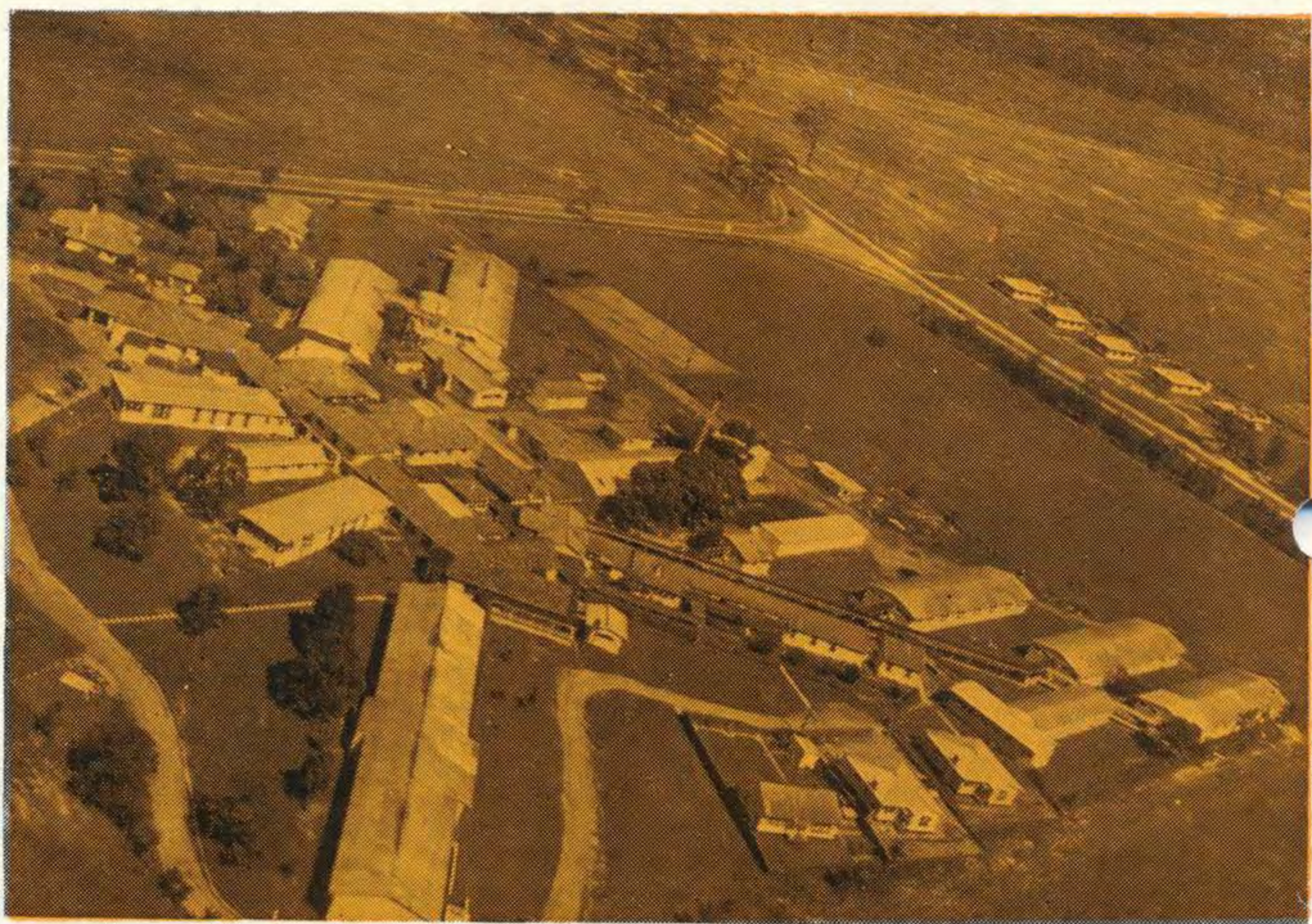
The new perimeter road slices across the paddocks near the Yallourn Hospital.
