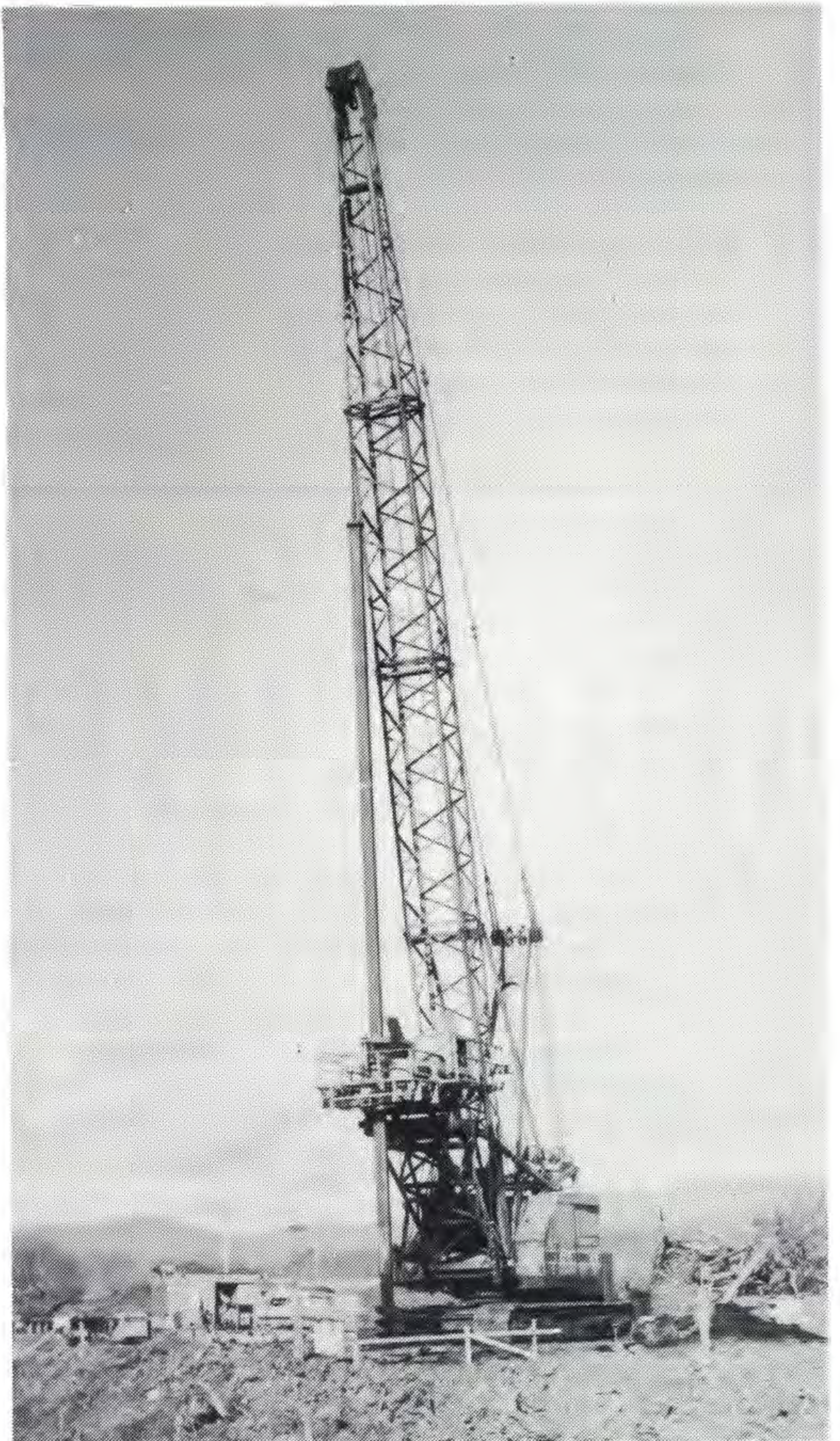
Work is underway on the $450,000 Mattingley Hill Road bridge at Traralgon South. A large crane (above) is currently drilling foundation holes for bridge Pylons.
