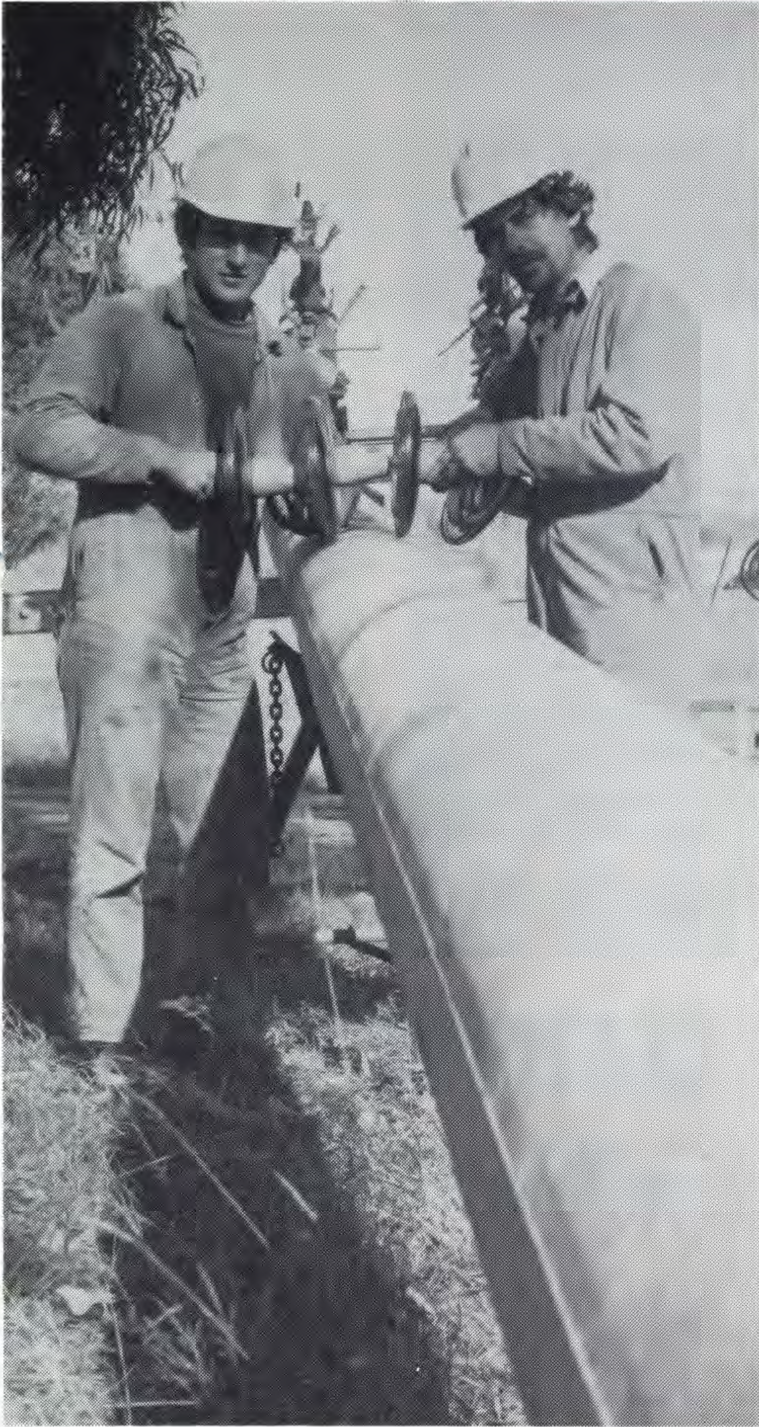
Linesman Mario Di Dio (left) and Linesman's assistant Francis Zonneveld get ready to attach an insulator to one of the new concrete poles, a number of which can now be seen on the new route between Morwell and Loy Yang.
