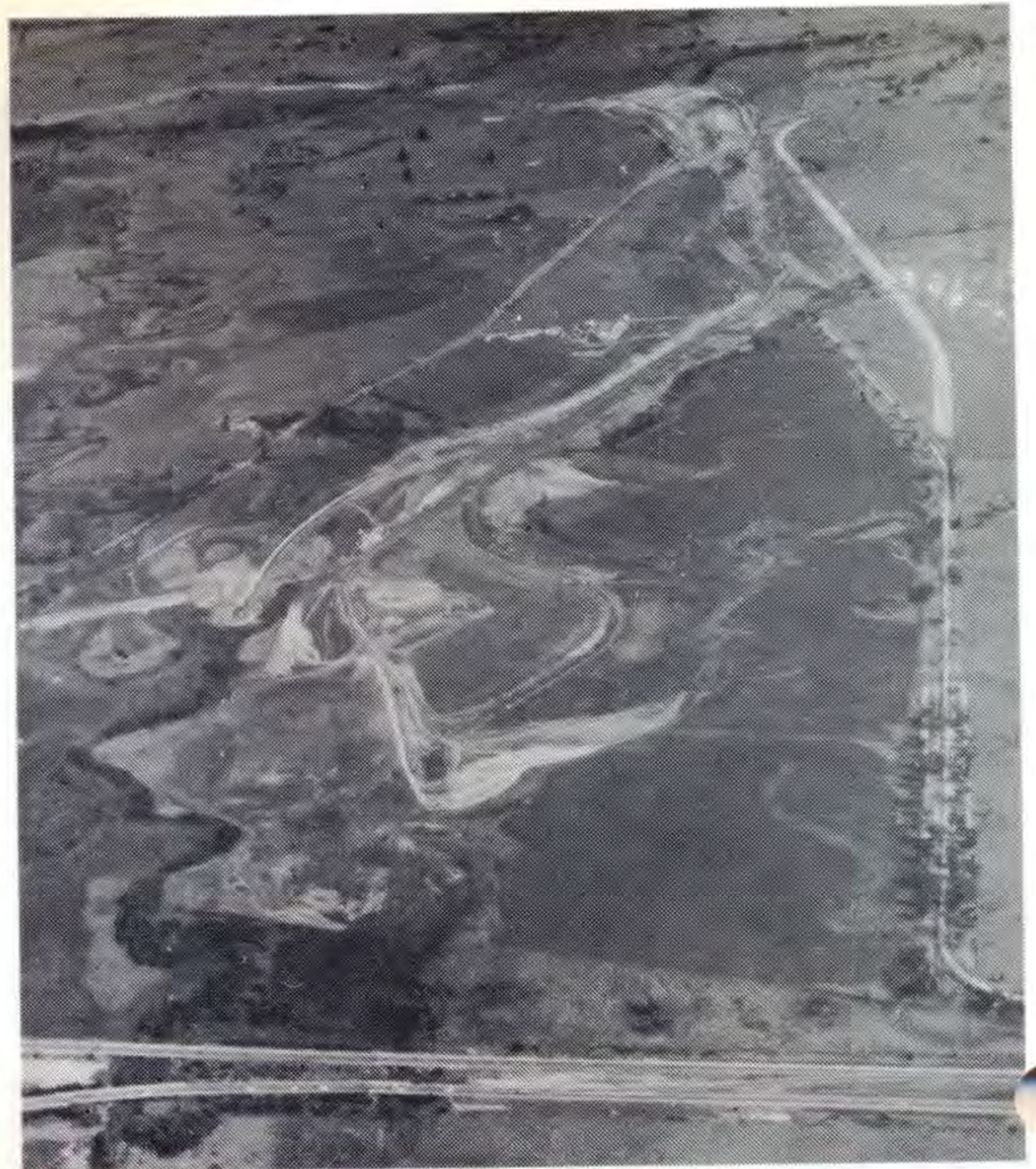
Above: This picture indicates the length of the Morwell River Diversion Project. It was taken before the heavy July rains and the flooding which followed — covering a large area.
