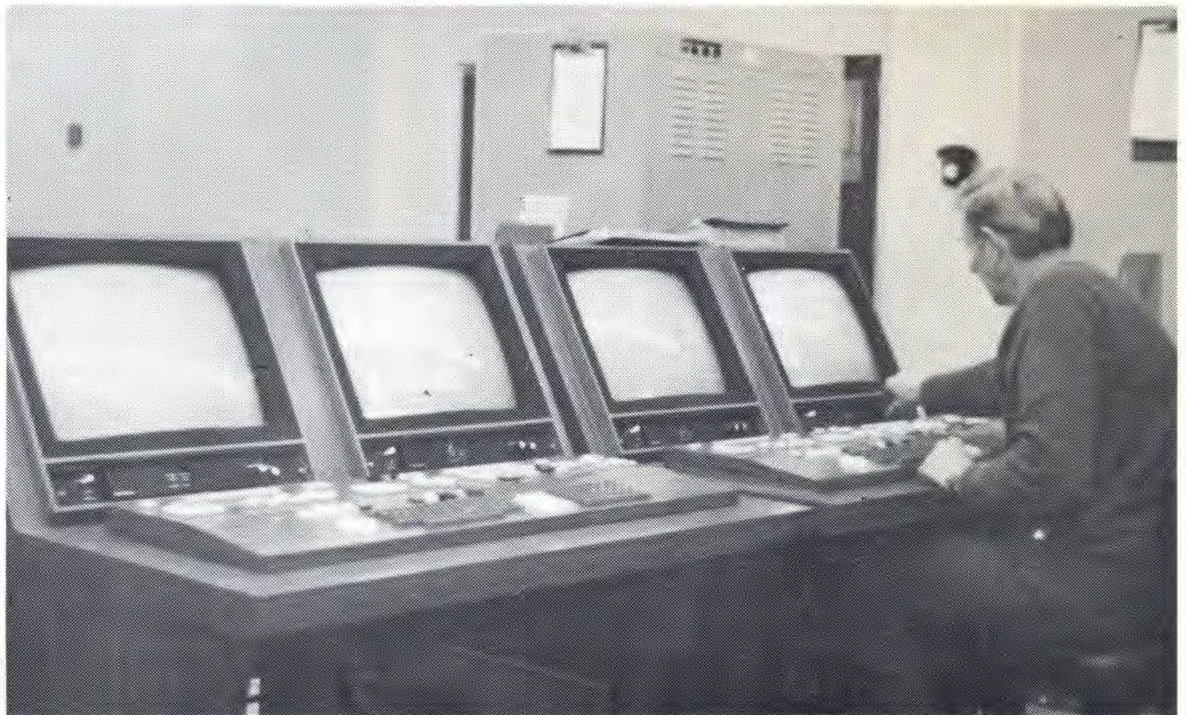
Above: Checking the new units in the Latrobe Valley Control Centre is Regional Control Officer (Procedures) Gavan Edmondson
