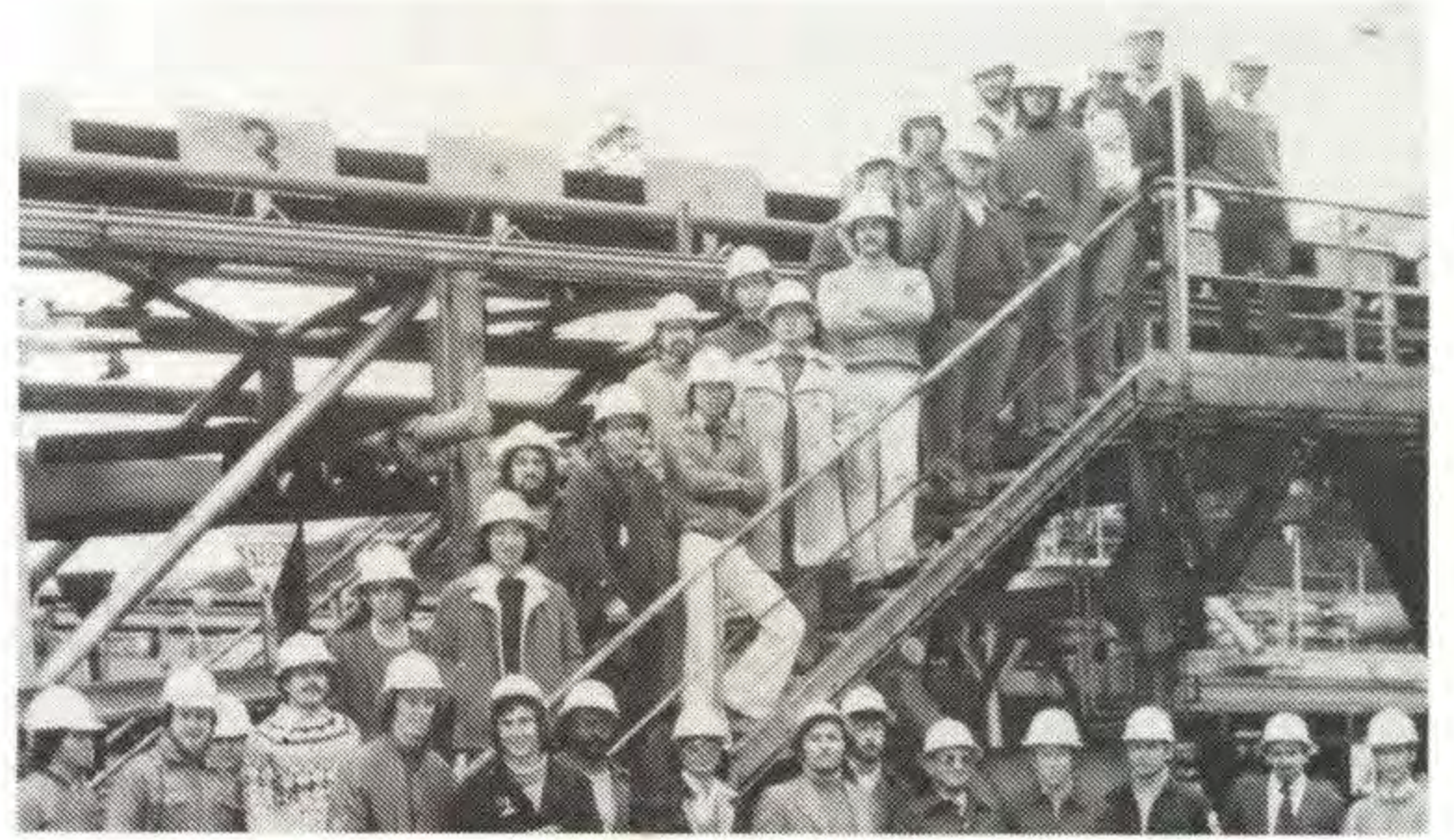
Pictured in front of a portion of the Morwell open cut conveyor system are final year power students from the University of New South Wales.
