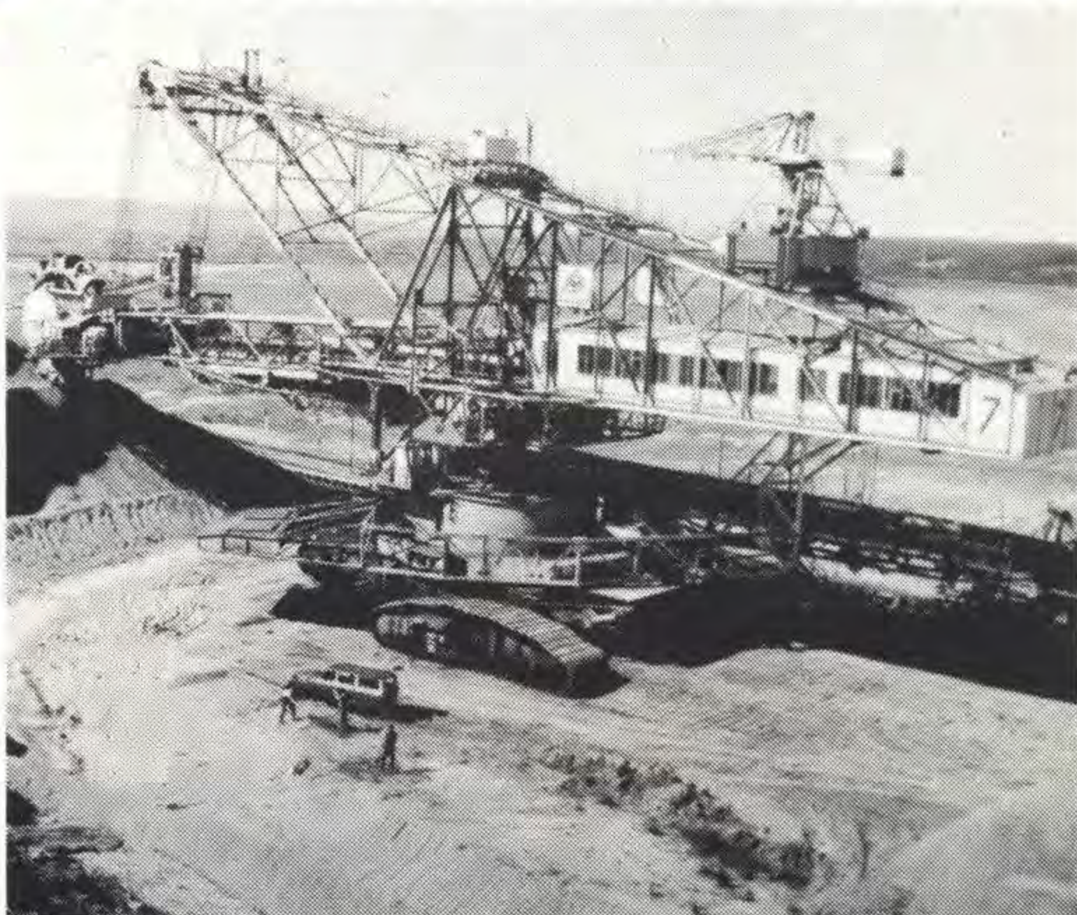
This picture of No. 7 dredger eating into overburden at Yallourn shows the easy way of getting rid of "bulges".
